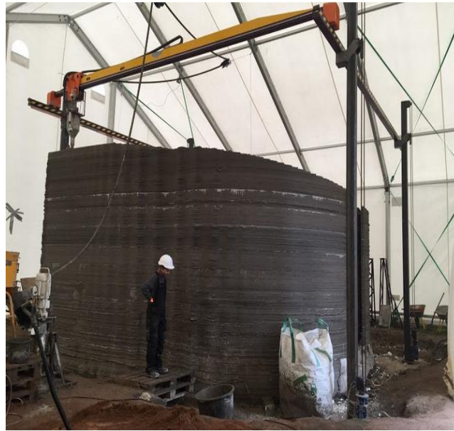
3D Printing of House with Smart materials
